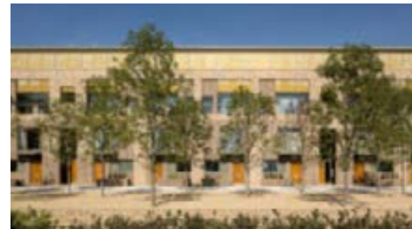
Figure 36: Great Kneighton, Cambridge – range of street types and scales with clear townscape markers and nodes created by varying building height (Proctor and Matthews)
