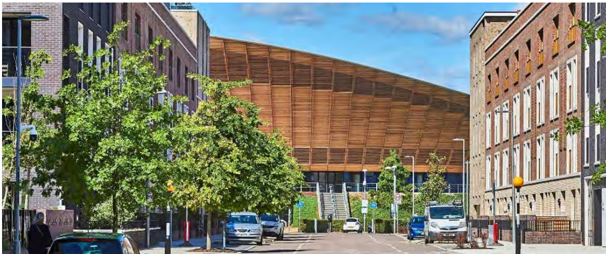
Figure 41: Chobham Manor, Olympic Park, London – wide mix of different housing types, including mews, terraces, multi-generational homes, duplexes, maisonettes and apartments (PRP)
